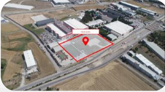
Photon Detector and Nanotechnology Facility
