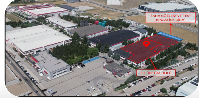
EO FLIR Systems Production Facility
